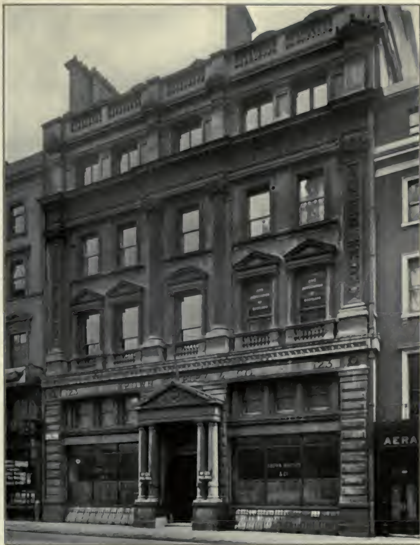
The London Office—Pall Mall
